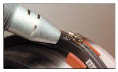
Stage 4: Cure epoxy adhesive with hot air gun.
